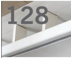
128 Metal Bulkhead RAM 5011-5012
